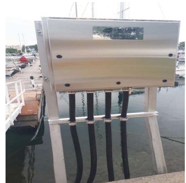
First stage complete.
