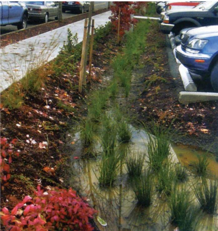
Bioswales can be used to maximize water infiltration and should be incorporated into the design of streets.
