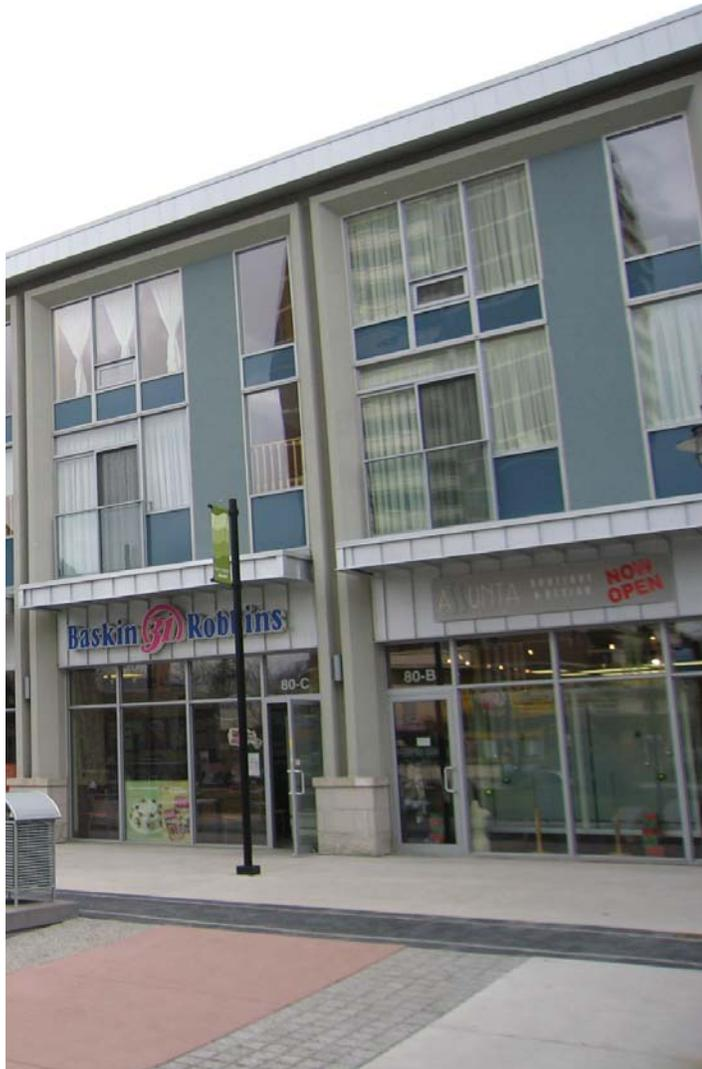
The ground floor of new mixed use commercial development should be taller (4.5 metres) to accommodate large windows, recessed entries and signage.
