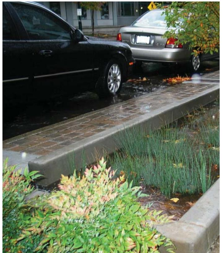
*Incorporating biofiltration trenches along the streetscape reduces the amount of impervious surfaces and run-off, and naturalizes the streetscape.*
