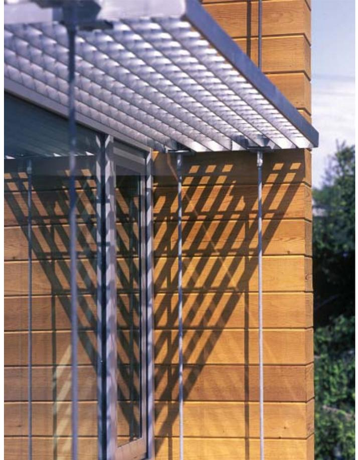
*Louvers control direct sunlight and maximize desirable indirect daylighting.*
