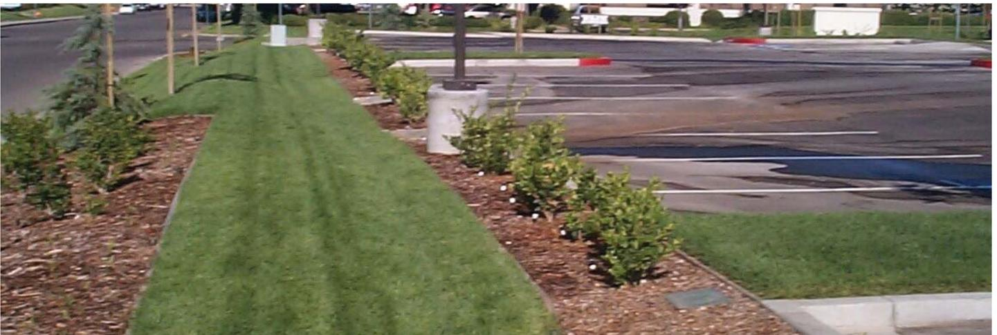
*This native, drought resistant landscaping reduces the impervious surface created by the adjoining parking lot. Rainwater is absorbed into the soil and minimizes the amount of discharge into the storm drain system.*
